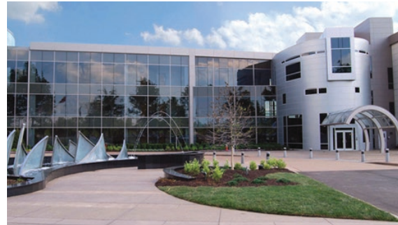
Parker Headquarters, Cleveland, Ohio, USA
