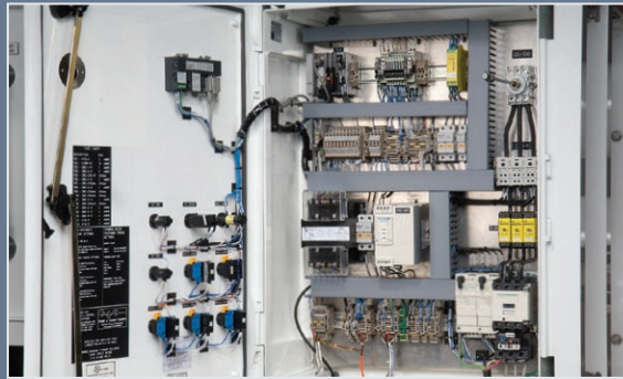
interior door / electrical
