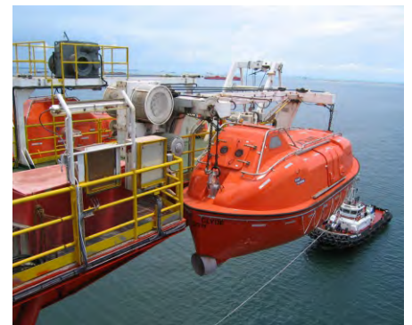
Platform Davit Installation
