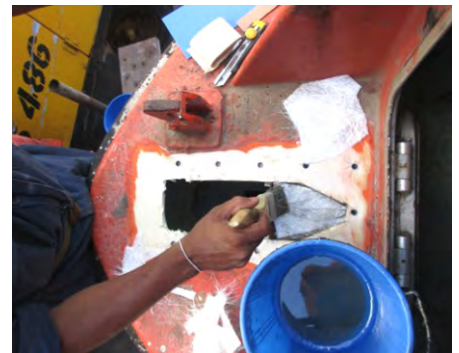
FRP Foundation Construction
