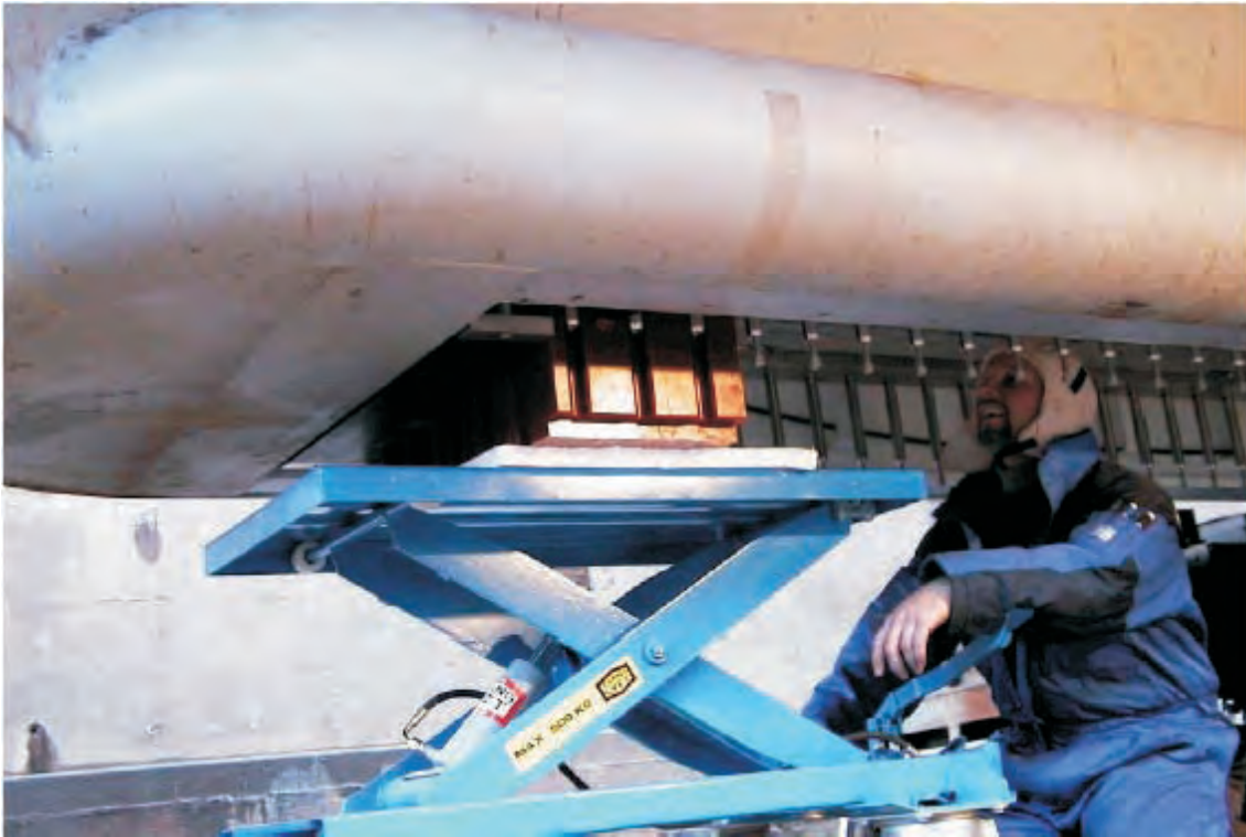
Figure 37 Flush installation blister for the EM 122
