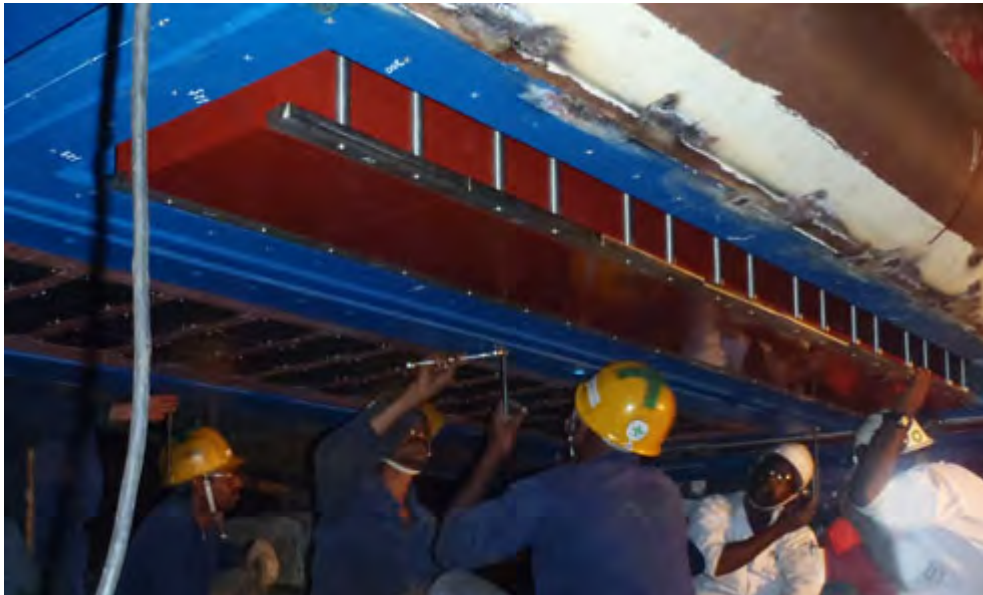
Figure 13 Transducer element installation EM 302
