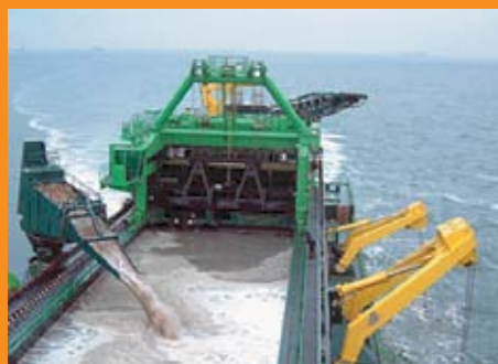
Stationary suction dredger
